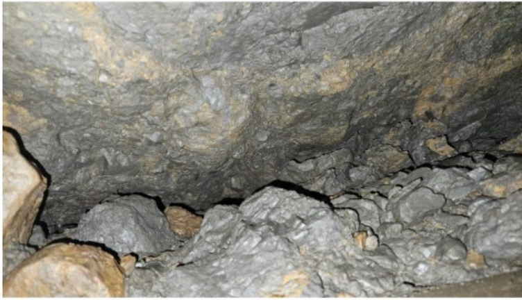
View above culvert crown looking downstream
