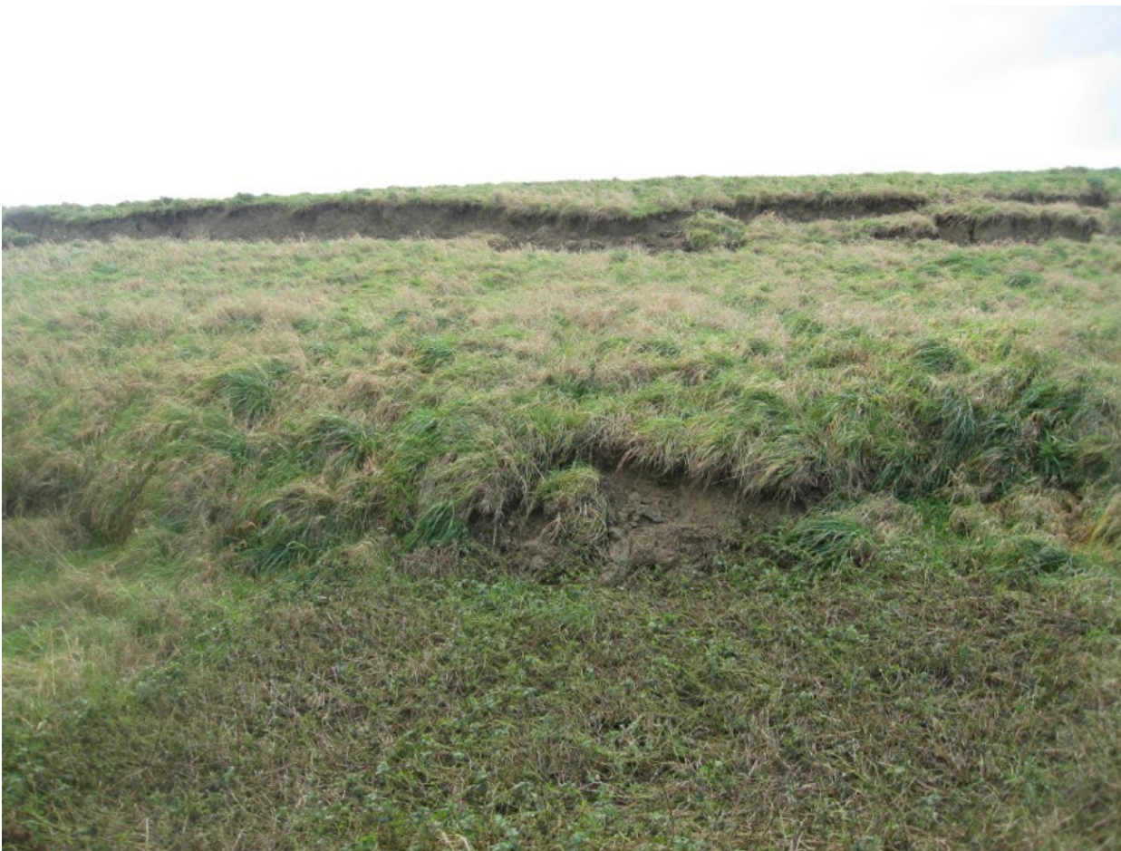
Longitudinal cracking of a thick topsoil layer on an embankment dam did not self heal, leading to a translational slip - Incident Image
