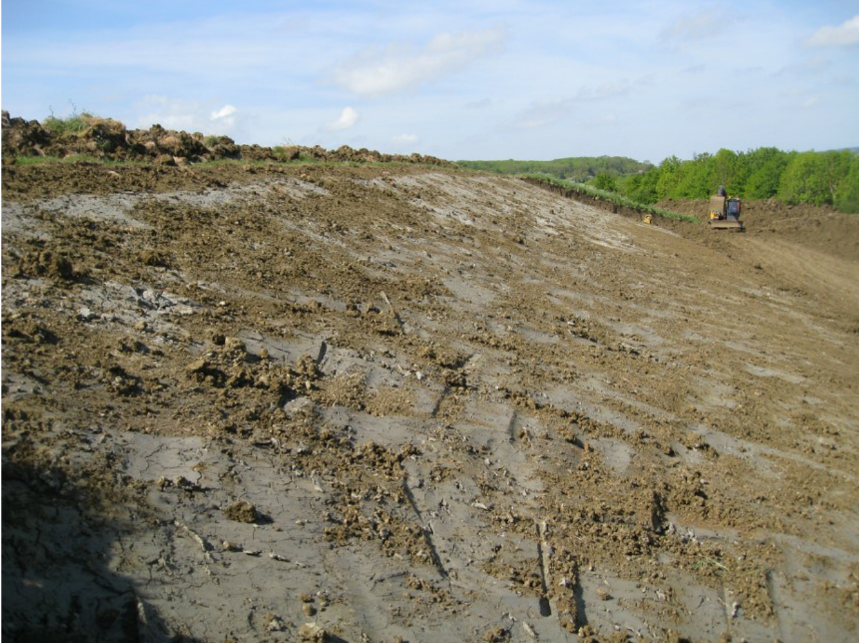
Longitudinal cracking of a thick topsoil layer on an embankment dam did not self heal, leading to a translational slip - Cause Image
