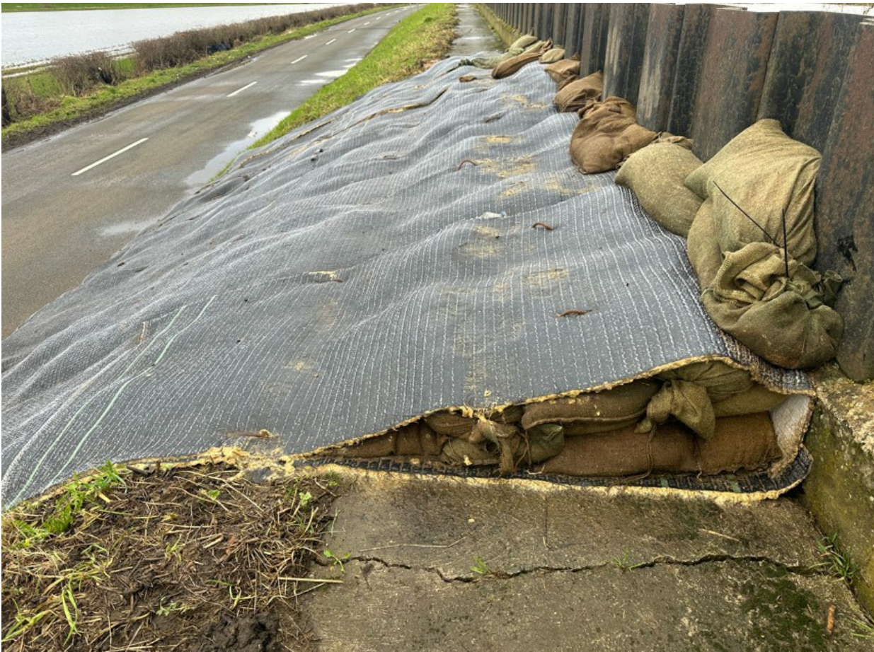
Erosion from overflowing of flood storage reservoir on embankment not designed to spill - Cause Image
