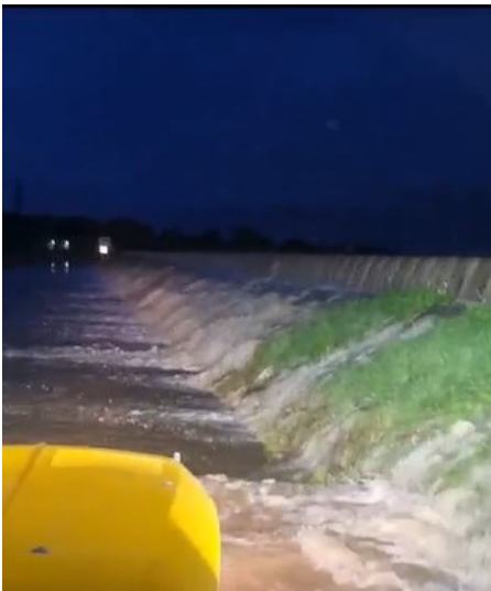
Erosion from overflowing of flood storage reservoir on embankment not designed to spill - Incident Image
