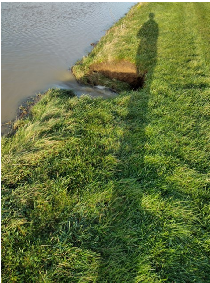
Leakage and breach of washland flood storage embankment - Incident Image
