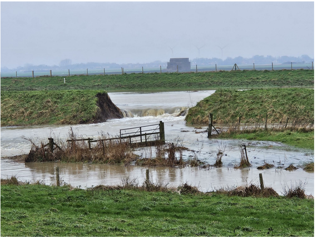
Leakage and breach of washland flood storage embankment - Incident Image
