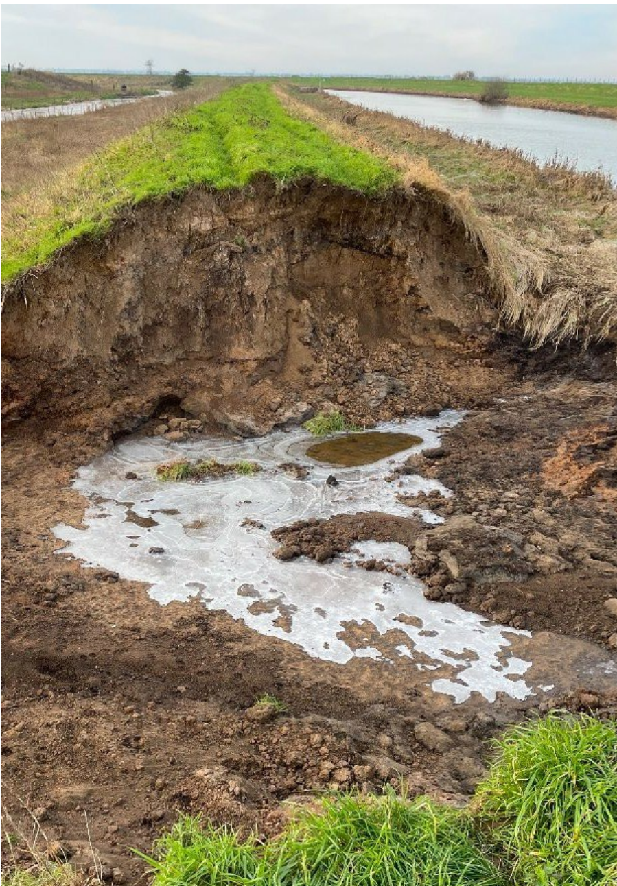
Leakage and breach of washland flood storage embankment - Incident Image
